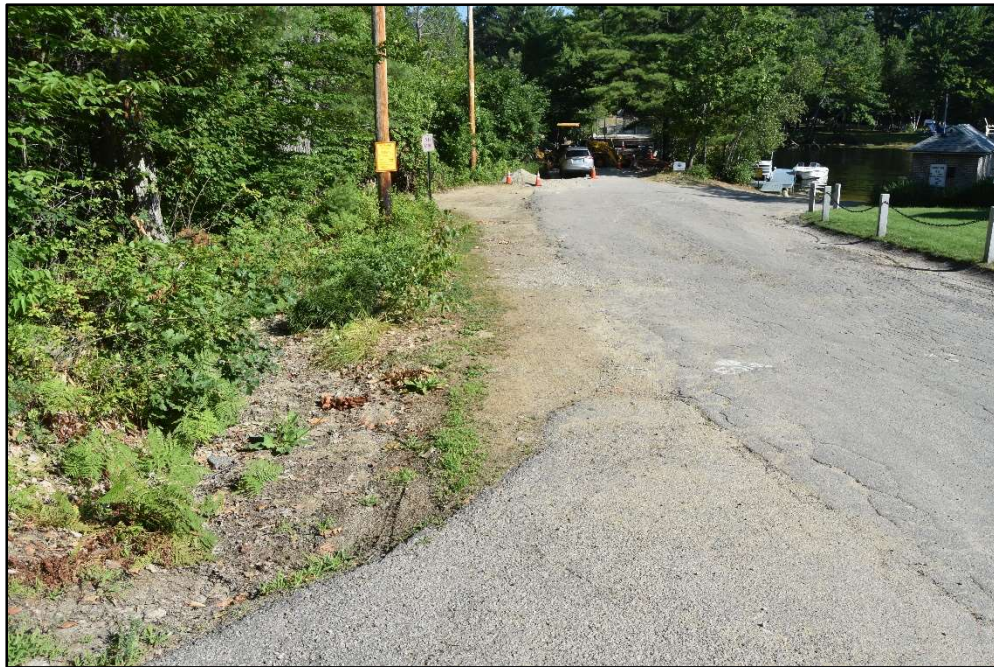
Figure 16. An example of graded surfaces along the road edge, view northwest.
