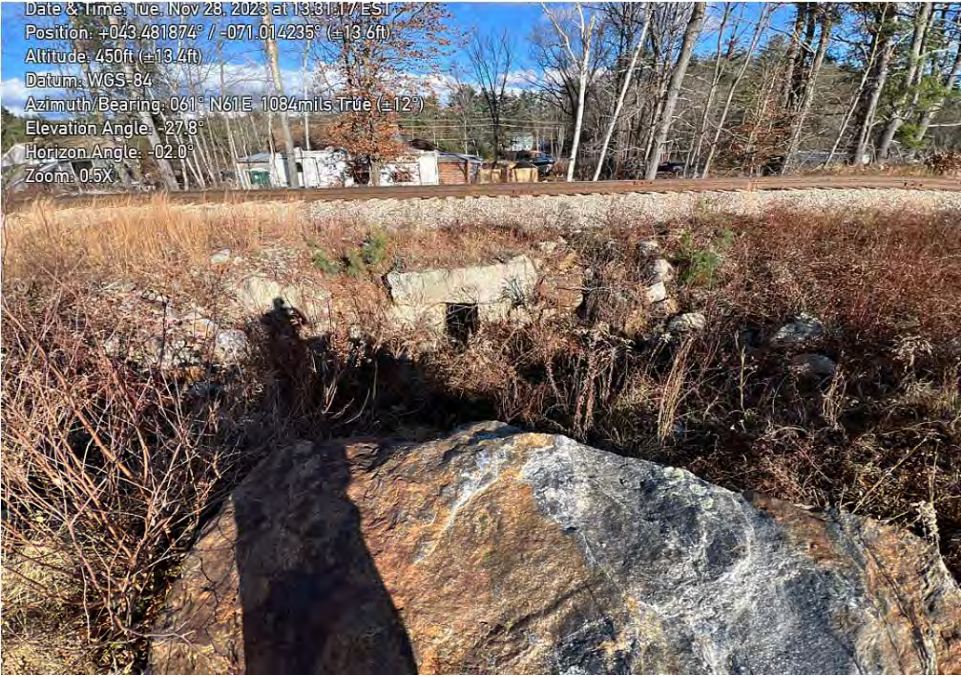
Really cool Rail Road Culvert.
