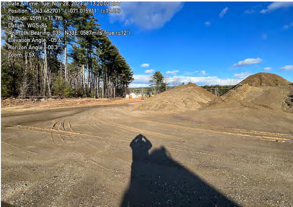
Material Storage looking at the administrative shed
