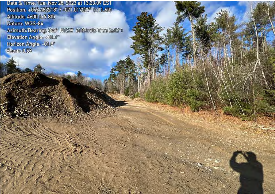
Main Pit Area at the easterly wood line, material storage.
