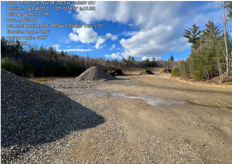
Access Road, material storage looking northwest into the mail pit.
