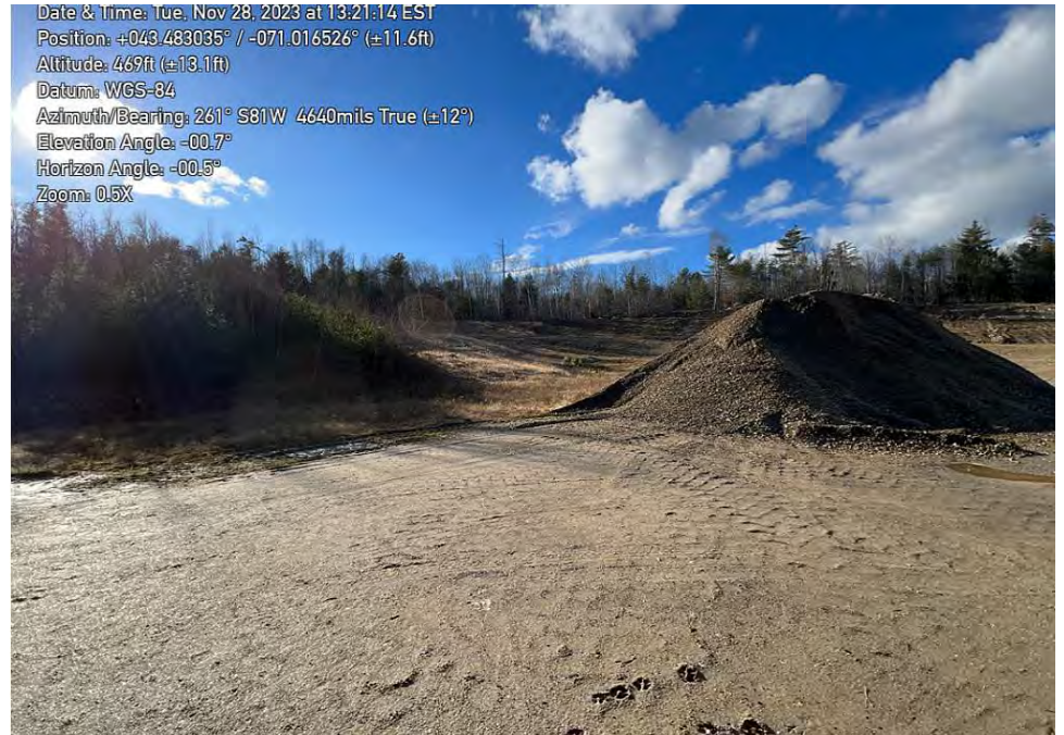
Main Pit Area, excavation floor and material storage
