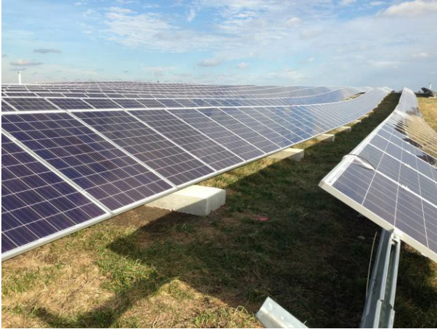
Ballasted system, showing distance between rows and the ballast blocks.
