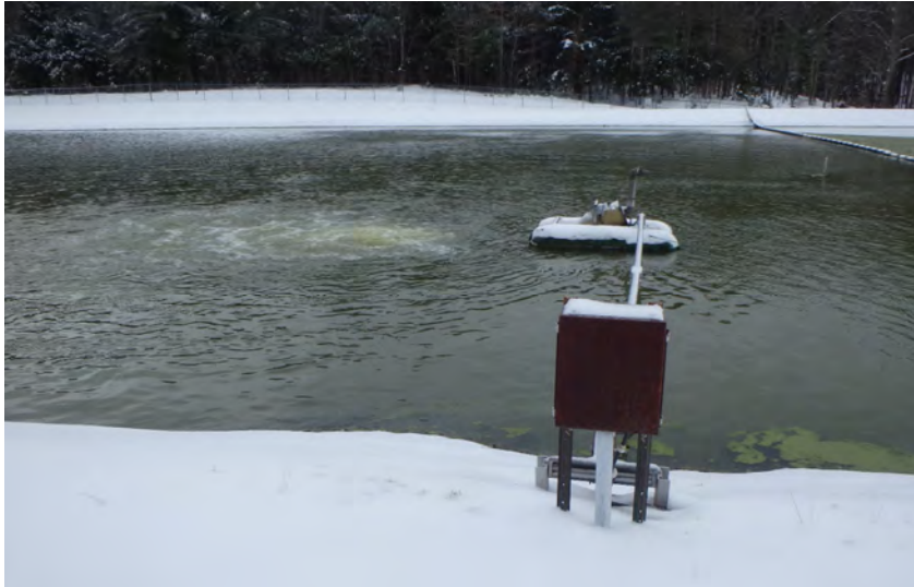
Lagoons with mechanical aerators
