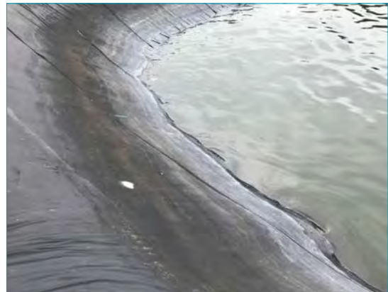
The lagoon liner shows significant signs of deterioration (below), which will be addressed as a part of this study.
